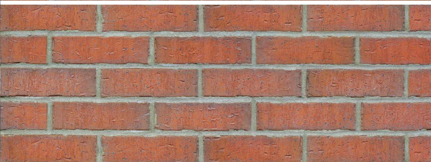
Brick tower HF03
